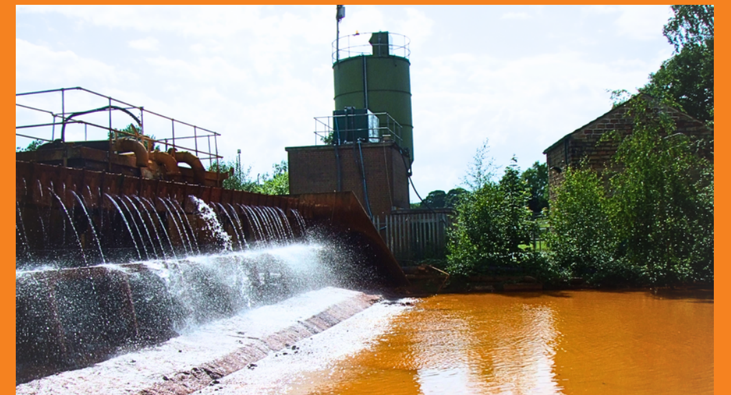
Water Flowing over the Weir on the Nature Trail
