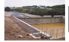
The water enters a balancing pond. It is orange because there are iron minerals in it from underground.
