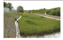
The water flows down again, into the reed beds, where the last of the iron particles stick to the reeds and only the clean water is allowed to flow into the stream.
